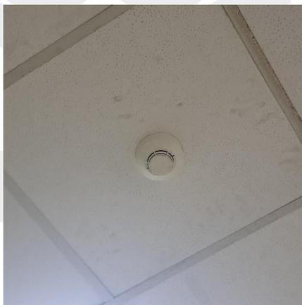
Gambar 4. 9 *Heat/smoke detection*
