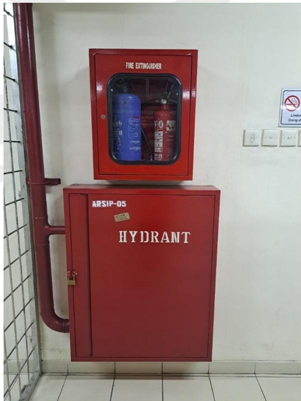
Gambar 4. 11 *Extinguisher & hydrant*
